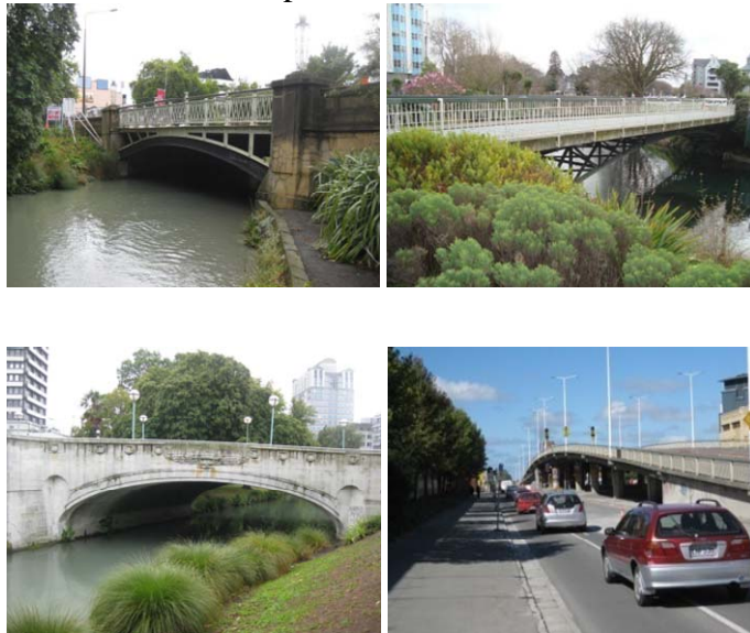
Figure 3. Selection of damaged bridges in the CBD area. Clockwise from top left: Colombo Street Bridge; Antigua Street Footbridge; Bridge of Remembrance; Moorhouse Avenue Overpass.
