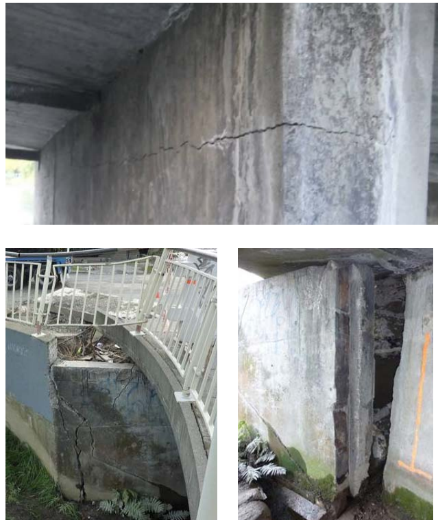
Figure 13. Gayhurst Road Bridge. (a) Damaged pier with flexural cracking [Photo by L. Hogan]; (b) Flexural cracks at the north-western wing-wall [Photo by L. Wotherspoon]; (c) Displacement of north-western wing-wall [Photo by L. Wotherspoon].
