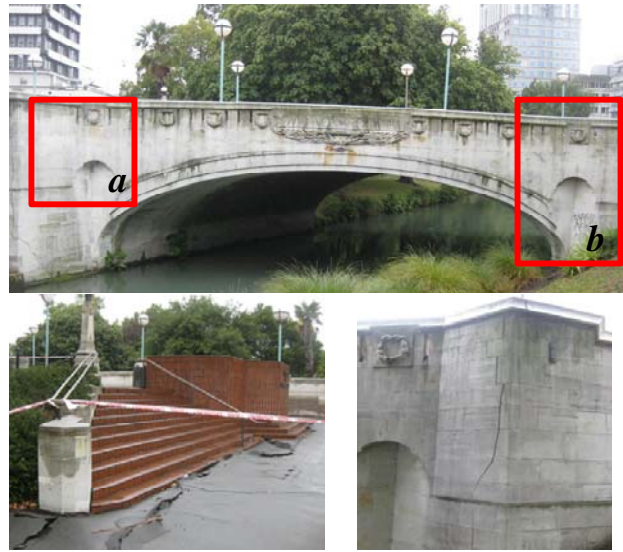
Figure 7. Bridge of Remembrance. (a) Damage to steps on western approach [Courtesy of OPUS]; (b) Damage to north-eastern wingwall [Courtesy of OPUS].
