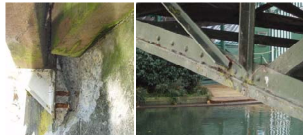
Figure 6. Antigua Street Footbridge. (a) Typical failure of end support to timber footway beams [Courtesy of OPUS]; (b) Typical failure of cross bracing member adjacent to corroded joint [Courtesy of OPUS].
