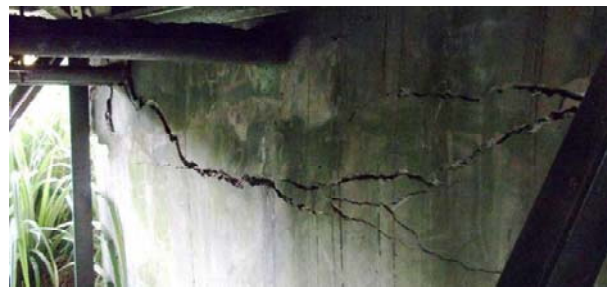
Figure 5. Antigua Street Footbridge. (a) View underneath showing hogging [Courtesy of OPUS]; (b) Damaged north-eastern abutment [Courtesy of OPUS].
