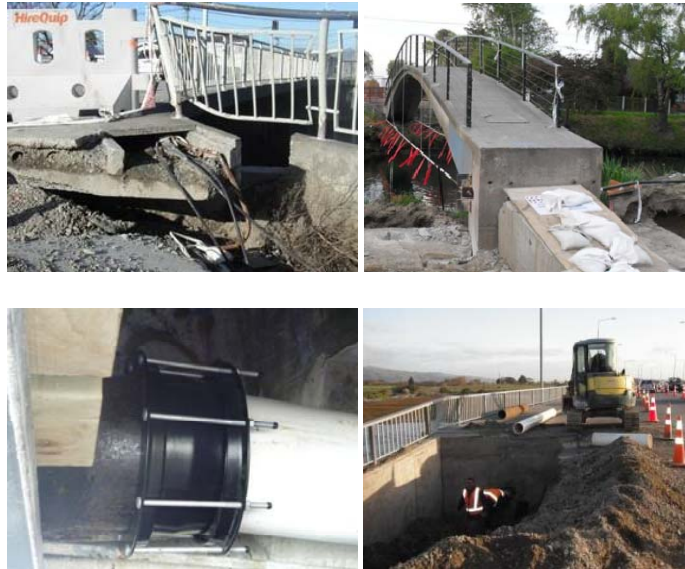
Figure 16. Damage to service lines. Clockwise from top left: Gayhurst Road Bridge: exposed lifelines [Photo by A. Palermo]; Dallington Pedestrian Footbridge: damage to electrical services to the Dallington area [Photo by M. Le Heux]; Repairing works at Bridge Street Bridge [Photo by A. Palermo]; Repair to water pipe at Bridge Street Bridge [Photos by A. Campbell].
