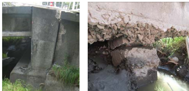
Figure 14. Fitzgerald Avenue Bridge. (a) Damage at the approach of the eastern bridge [Photo by Anton Kivell]; (b) Back rotated abutments [Courtesy of OPUS]; (c) Flexural cracks on the piles [Photo by L. Hogan].
