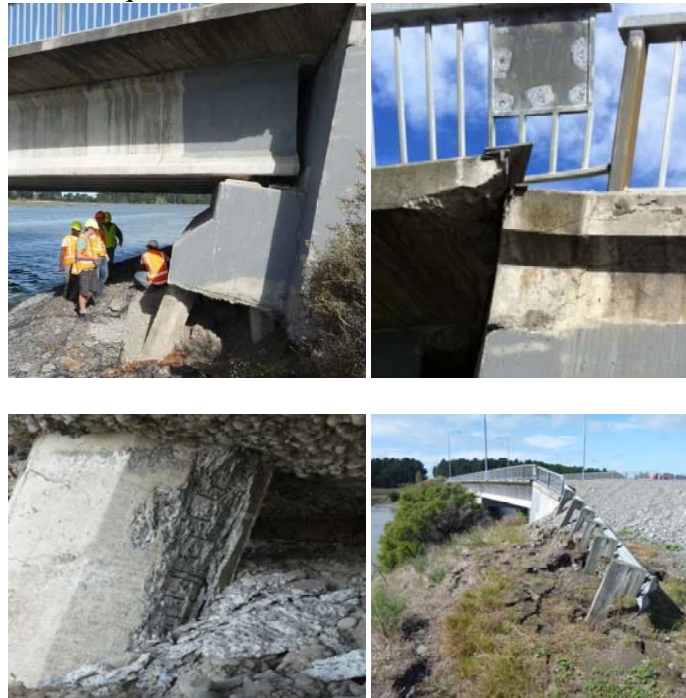
Figure 12. Bridge Street Bridge. Clockwise from top left: Back rotated abutments [Photo by M. Bruneau]; pounding of the deck on the abutment [Photo by A. Kivell]; West approach settlement and temporary repair [Photo by S. White]; plastic hinging in abutment piles of Bridge Street Bridge [Photo by M. Bruneau].
