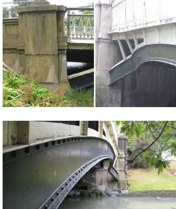
Figure 4. Colombo Street Bridge. Clockwise from top left: rotation of the abutment [Courtesy of OPUS]; buckling of steel arch [Photo by M. Yashinsky]; close up view of the steel arch [Courtesy of OPUS].
