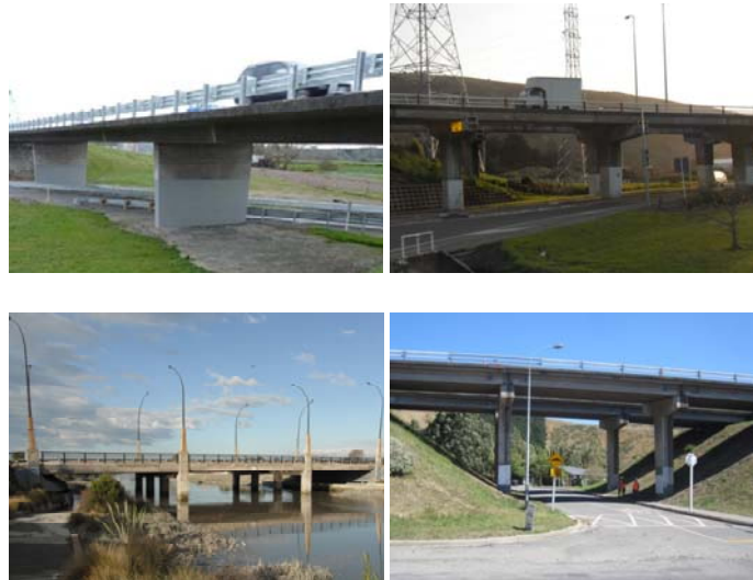
Figure 15. Overall view of some damaged highway bridges after February 22, 2011. Clockwise from top left: Chaney's Overpass [Photo by M. Anagnostopoulou]; Port Hills Overbridge [Courtesy of OPUS]; Horotane Overbridge [Courtesy of OPUS]; Anzac Drive Bridge [Photo by E. Camnasio] [Palermo et al. 2011a].
