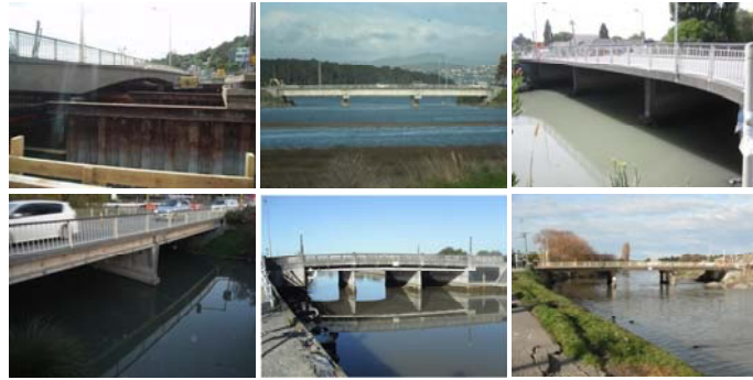
Figure 10. Selection of damaged road bridges. Clockwise from top left: Ferrymead Bridge; Bridge Street Bridge; Gayhurst Road Bridge; Avondale Road Bridge; Pages Road Bridge; Fitzgerald Avenue Bridge.
