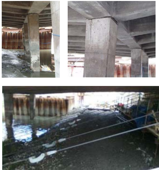
Figure 11. Ferrymead Bridge. (a) Tilted piers [Courtesy of OPUS]; (b) Close-up view of flexural cracks at the top of the piers [Courtesy of OPUS]; (c) Securing works of Ferrymead Bridge [Courtesy of OPUS].
